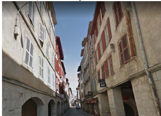
c) Inside view of the street.
